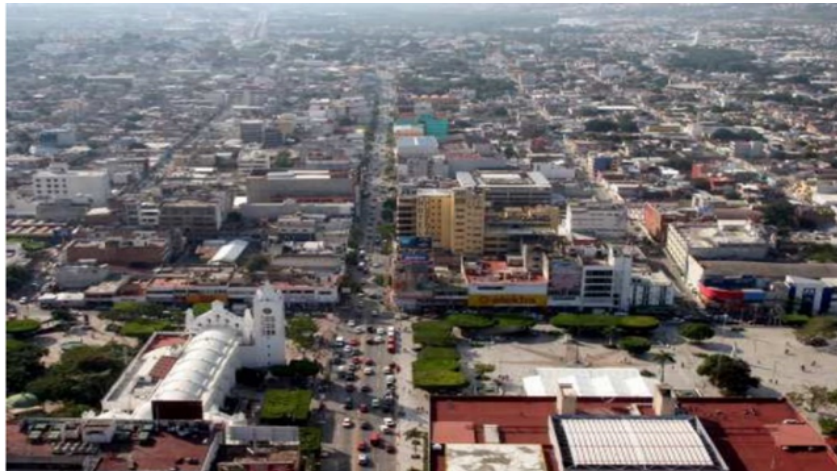
Figure 1. City of Tuxtla Gutiérrez, roof diversity. Source: Photo by Chiapas Paralelo
