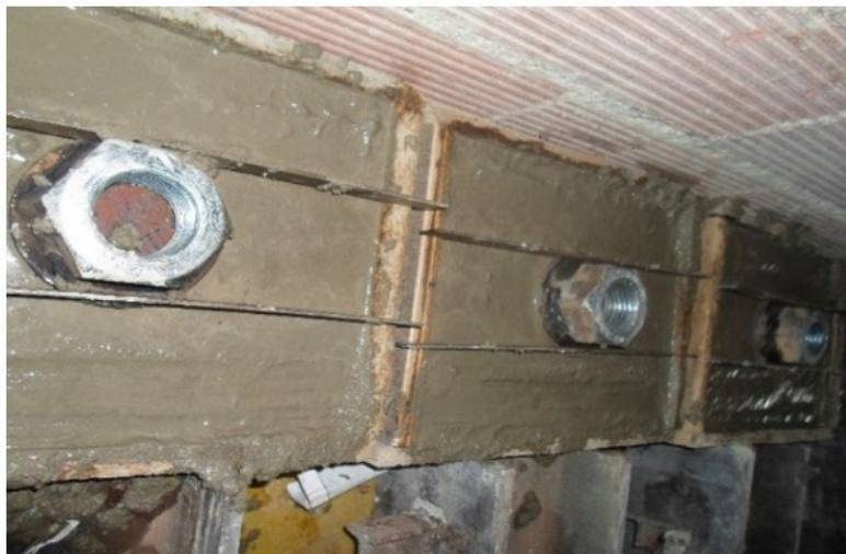
Figure 3. Concrete pouring of specimens.
