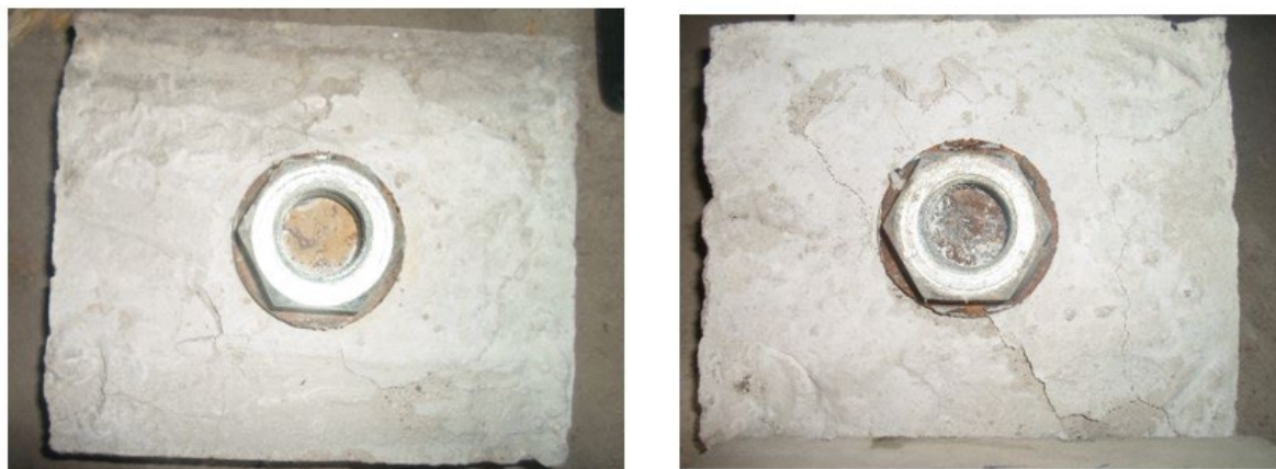
Figure 9. Concrete failure for IPE6N, IPE8N.
