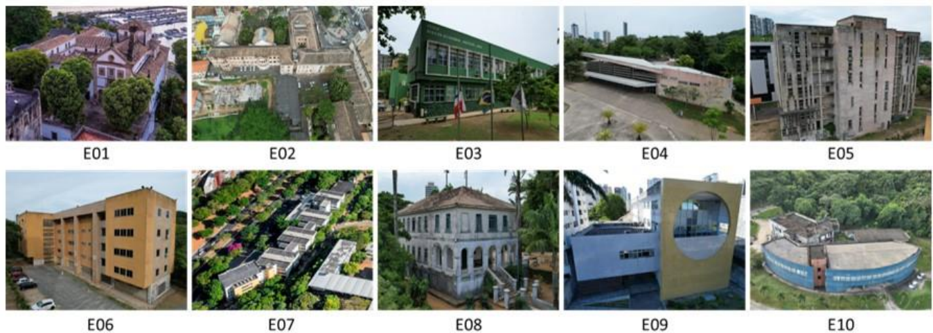
Figure 2. Representative images of inspected buildings.
